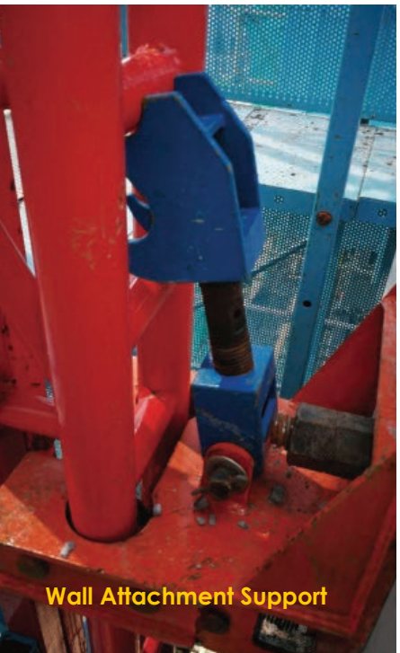
Connection between Horizontal Trusses and Vertical Poles
